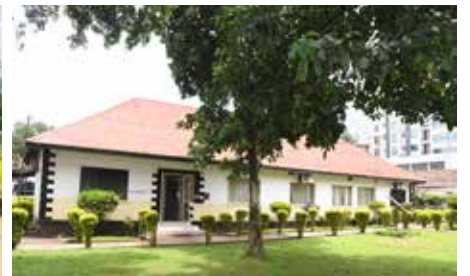
Jengo lililoboreshwa-TVLA Arusha
